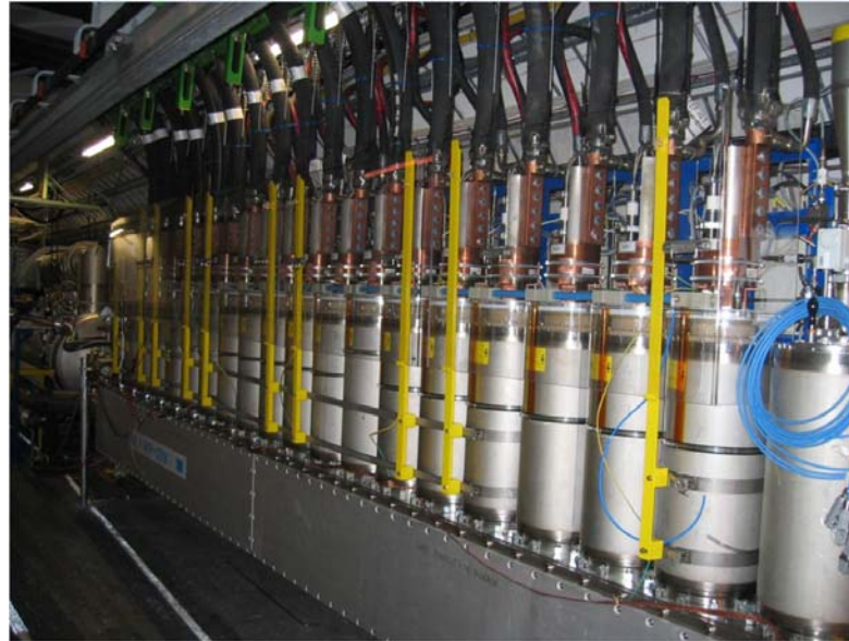
New "DFB": joint box
